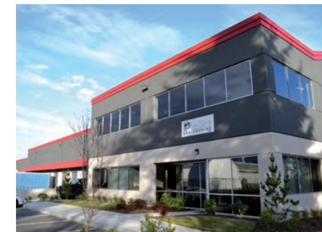
New assembly facility in 2510 West Casino Road, in Everett ( USA).
