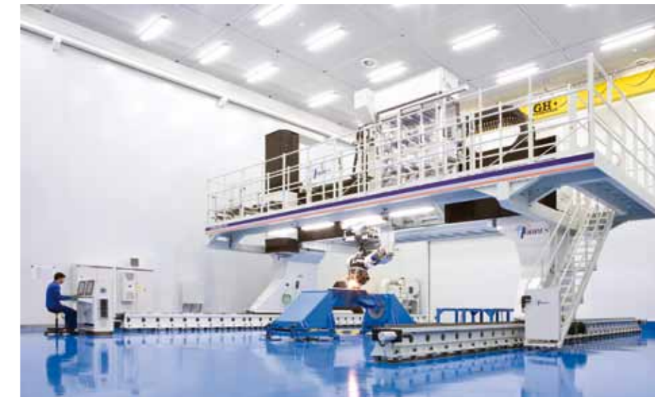
Clean room overview.
